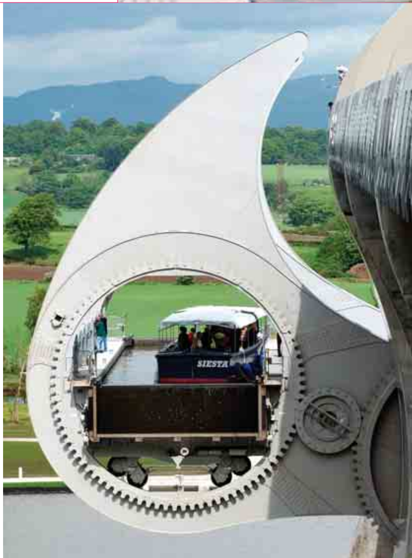
A rotating caisson in operation
