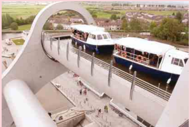
A tour boat sailing through an aqueduct at the top of the lift
