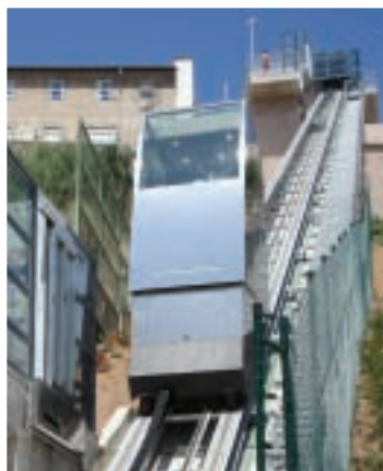
View of auxiliary escalator
